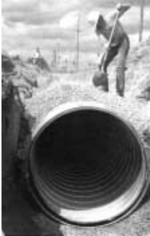
Spiral rib pipe installation.
