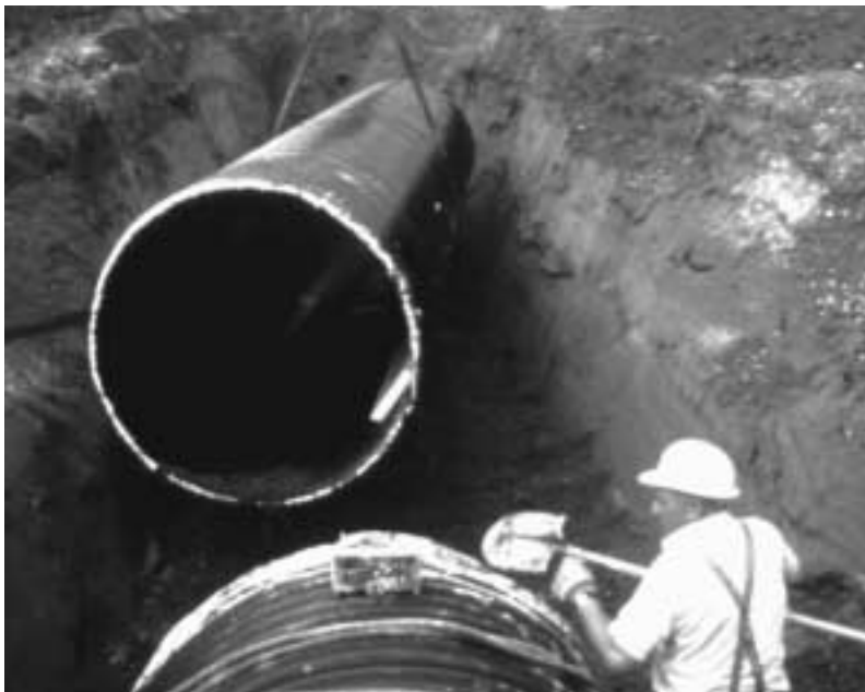
Placing coated CSP sewer section. Fabric sling protects pipe coating.
